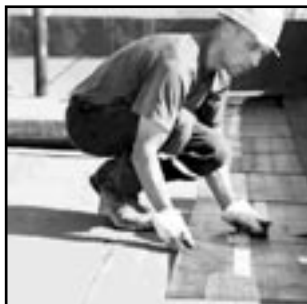
FLAT TOP ROOF
