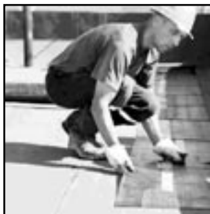
FLAT TOP ROOF
