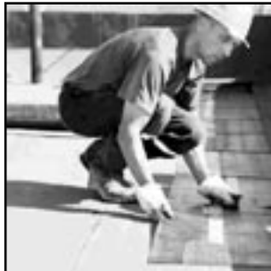
FLAT TOP ROOF
