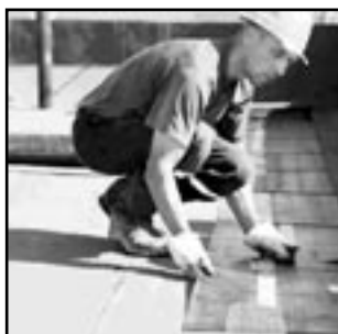
FLAT TOP ROOF
