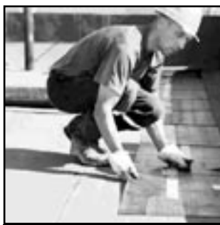
FLAT TOP ROOF
