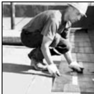
FLAT TOP ROOF
