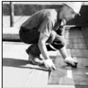
FLAT TOP ROOF
