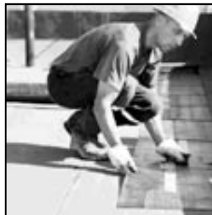
FLAT TOP ROOF
