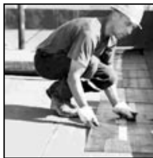
FLAT TOP ROOF
