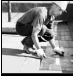
FLAT TOP ROOF
