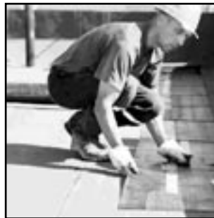
FLAT TOP ROOF
