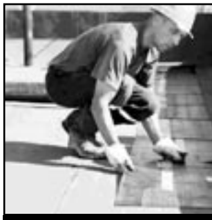
FLAT TOP ROOF
