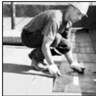
FLAT TOP ROOF
