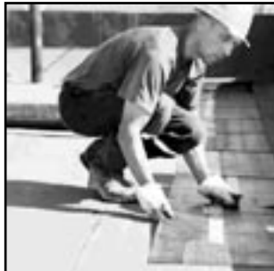
FLAT TOP ROOF
