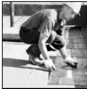
FLAT TOP ROOF
