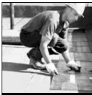
FLAT TOP ROOF
