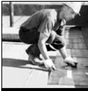
FLAT TOP ROOF
