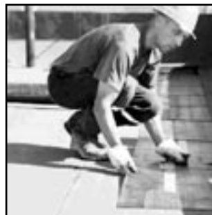
FLAT TOP ROOF
