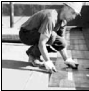
FLAT TOP ROOF
