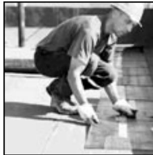
FLAT TOP ROOF
