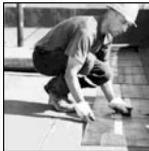
FLAT TOP ROOF
