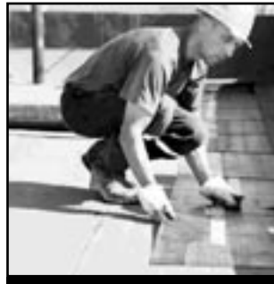
FLAT TOP ROOF
