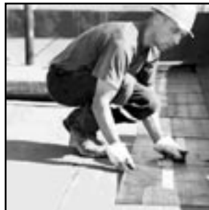
FLAT TOP ROOF
