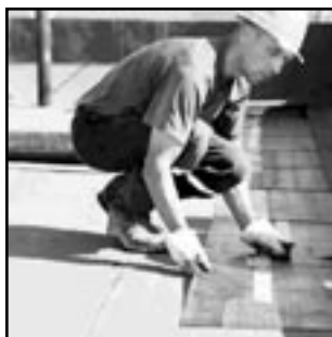
FLAT TOP ROOF
