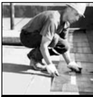
FLAT TOP ROOF
