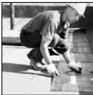
FLAT TOP ROOF
