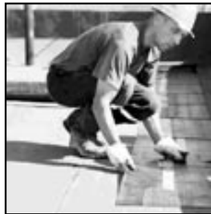
FLAT TOP ROOF
