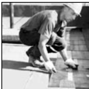
FLAT TOP ROOF
