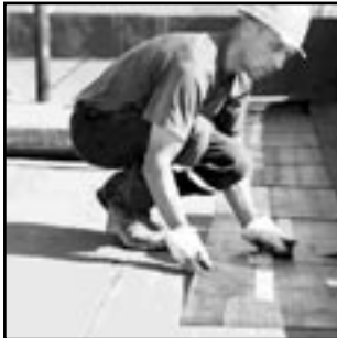
FLAT TOP ROOF
