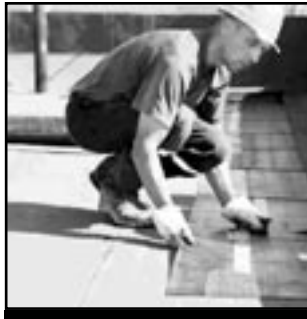
FLAT TOP ROOF
