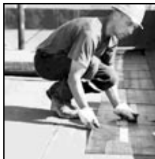
FLAT TOP ROOF
