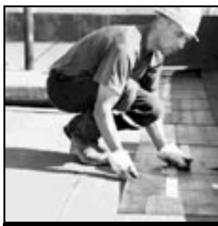
FLAT TOP ROOF
