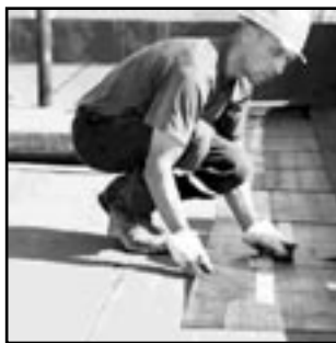
FLAT TOP ROOF
