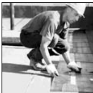
FLAT TOP ROOF
