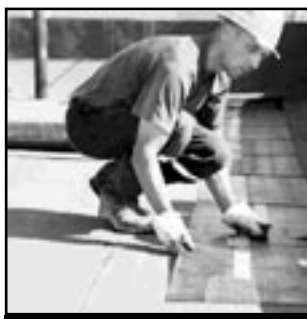
FLAT TOP ROOF
