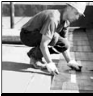
FLAT TOP ROOF
