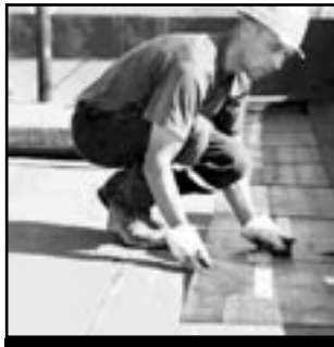
FLAT TOP ROOF
