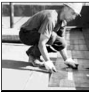
FLAT TOP ROOF
