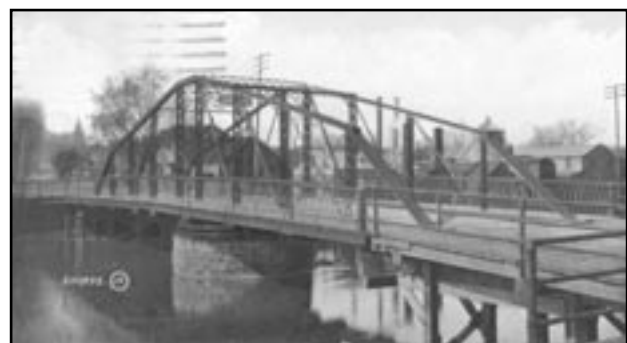
(above) After the Milton Avenue Draw Bridge was destroyed during the 1882 flood, this steel bridge was built. An overhead sign in the middle of the bridge read "Walk your horse or pay the fine." The brick support under the bridge remains to this day and supports the present bridge which was reconstructed in 2001.
