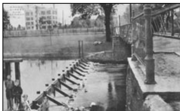
(above) Photo (circa 1914) shows the Grand Avenue Bridge when it was a truss bridge. The small dam was built in 1912 to keep the river at a depth that would allow for swimming and rowboats. The concrete arch bridge that stands today was built in 1917. Note the Wheatena building at top left.
