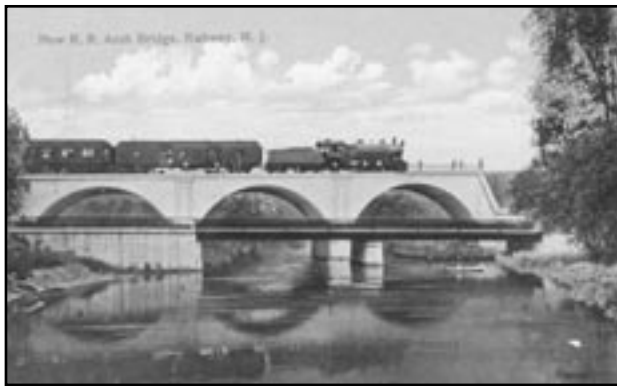
(above) A railroad bridge was constructed over the river in the 1830s when tracks were first laid in Rahway. In 1875 an iron bridge was built. It was reported to be the first four track iron bridge built in the United States. When the tracks were elevated (1911-1914) this new 3-arch concrete bridge was constructed.
