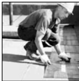
FLAT TOP ROOF
