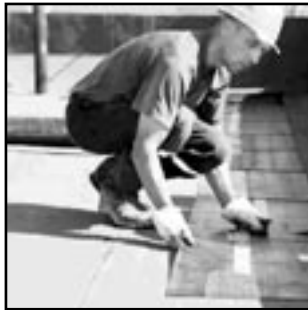
FLAT TOP ROOF
