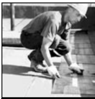
FLAT TOP ROOF
