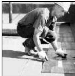
FLAT TOP ROOF
