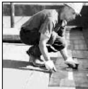
FLAT TOP ROOF
