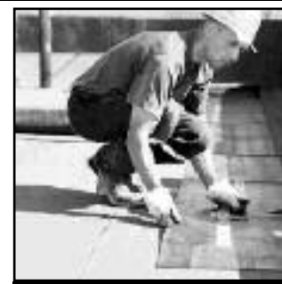
FLAT TOP ROOF
