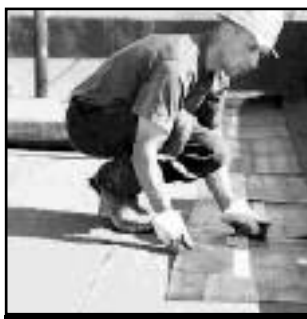
FLAT TOP ROOF
