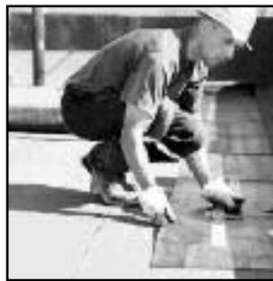
FLAT TOP ROOF
