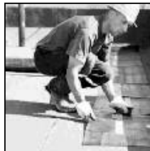
FLAT TOP ROOF
