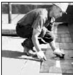
FLAT TOP ROOF
