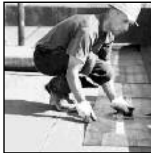
FLAT TOP ROOF
